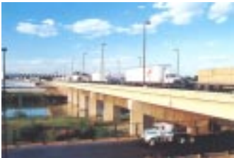
International Bridge II connecting Laredo, Texas and Nuevo Laredo, Tamaulipas, Mexico.
