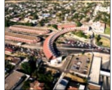
Laredo logs over 46,000 vehicular crossings daily.
