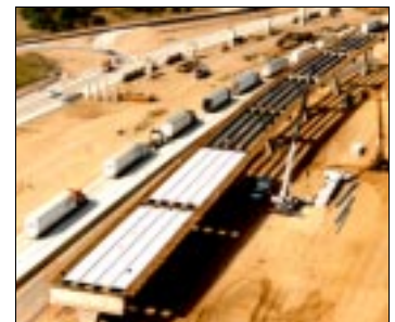
Construction of fly-over facilitating access to the World Trade Bridge.
